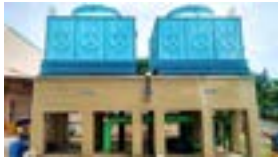
FRP COOLING TOWER
